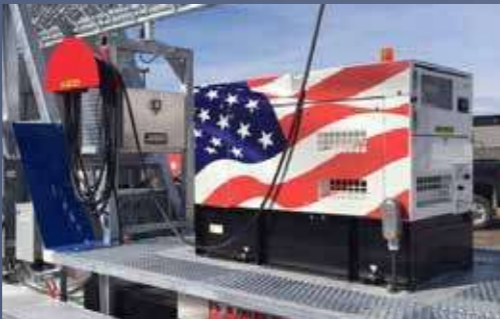
USA, Construction site
