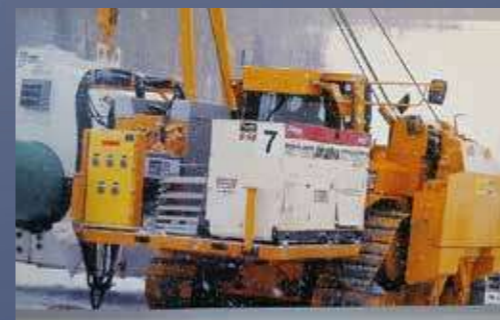
Russia, Construction site
