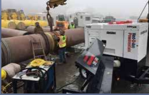
USA, Pipeline construction
